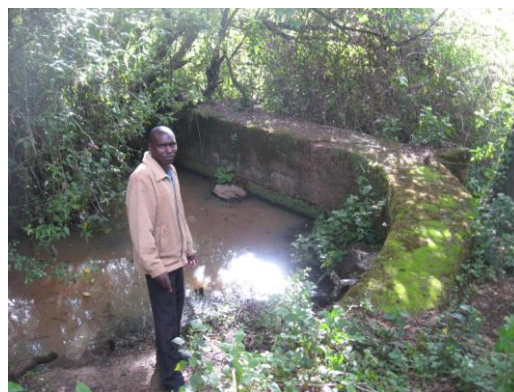
Old walls to spring in the hills
