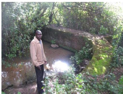
Old walls to spring in the hills
