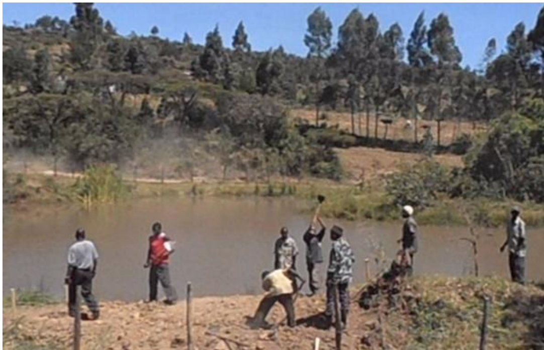
Ground Breaking for the Water Project
