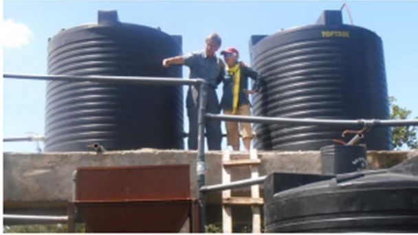
Joanne and Bill atop water purification plant at Kongasis
