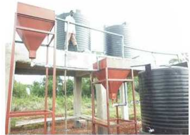
Stage three of the project. Water Purification via a two-stage Filtering process
